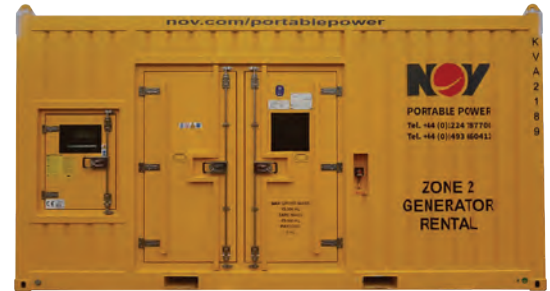
Containerised Zone 2 200kVA generator
