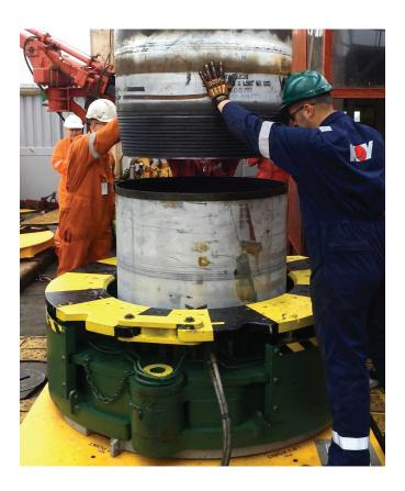
The only other alternative to XLC-S-HS was to weld the conductor pipe ends together as the string was run in the water. The biggest downside to welding pipe on the rig is time – with NDE (non-destructive examination), the estimated time it takes per joint is 3.5 to 4 hours. In comparison, the XLC-S-HS took an average of 6.82 minutes per connection to make-up.
