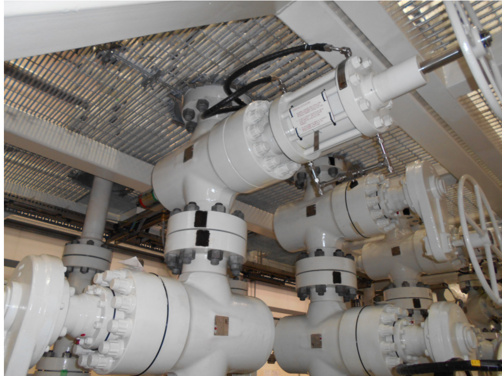
Anson E-Type with DA actuator and manual override built into an NOV choke and kill manifold for drilling application.
