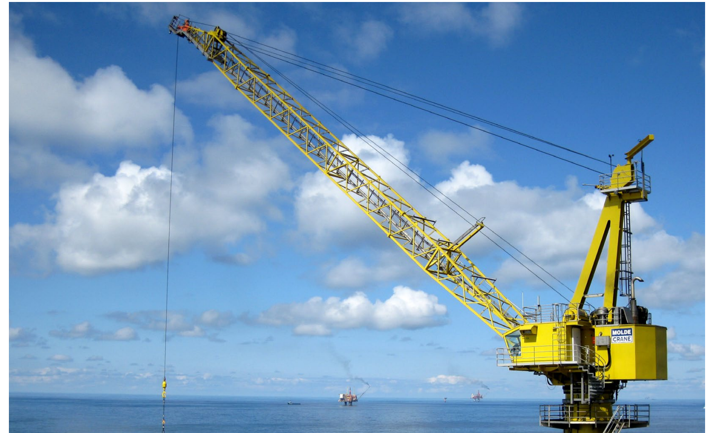
50 t crane on Statfjord B
