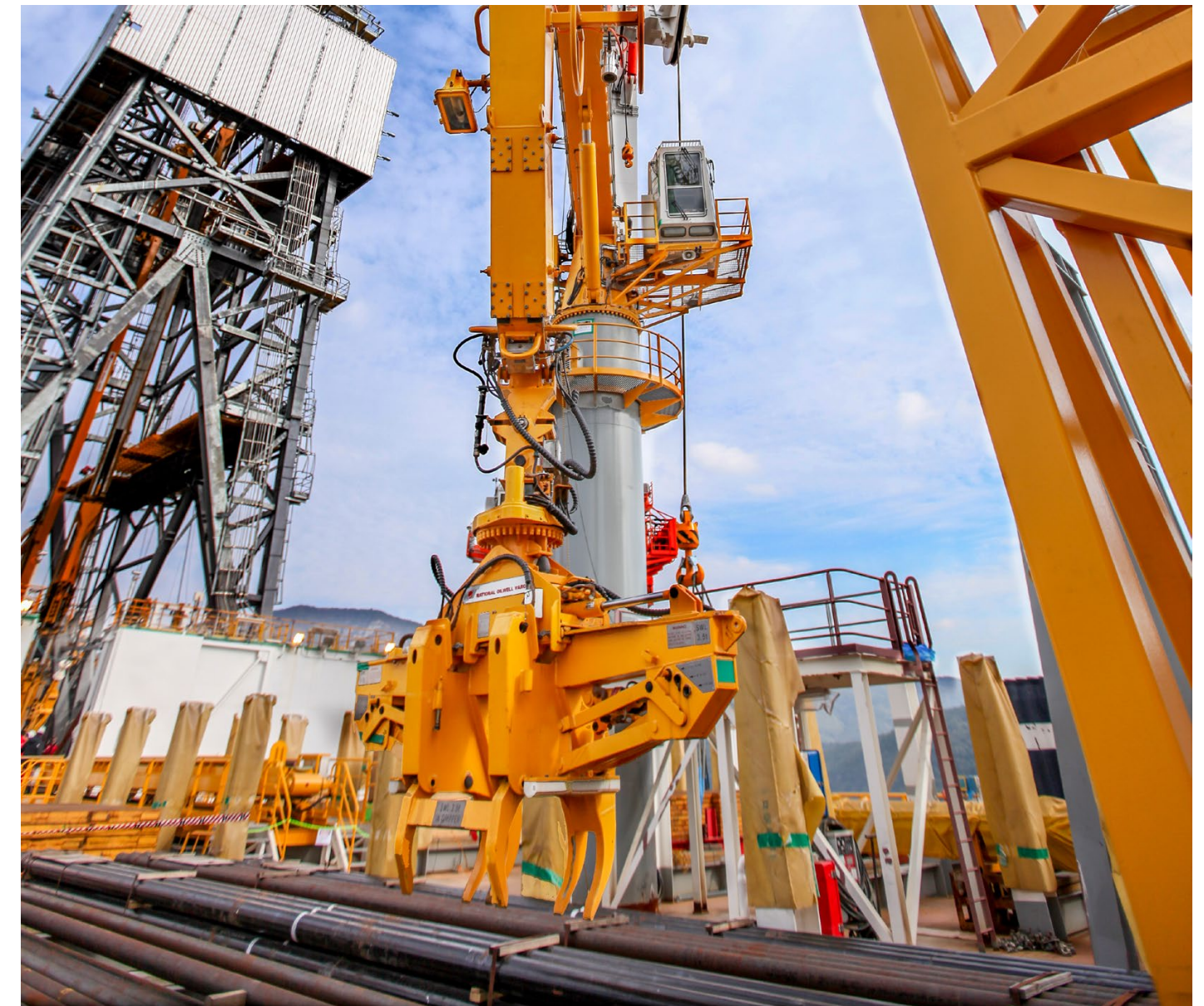
Pipehandling Crane on Drillship
