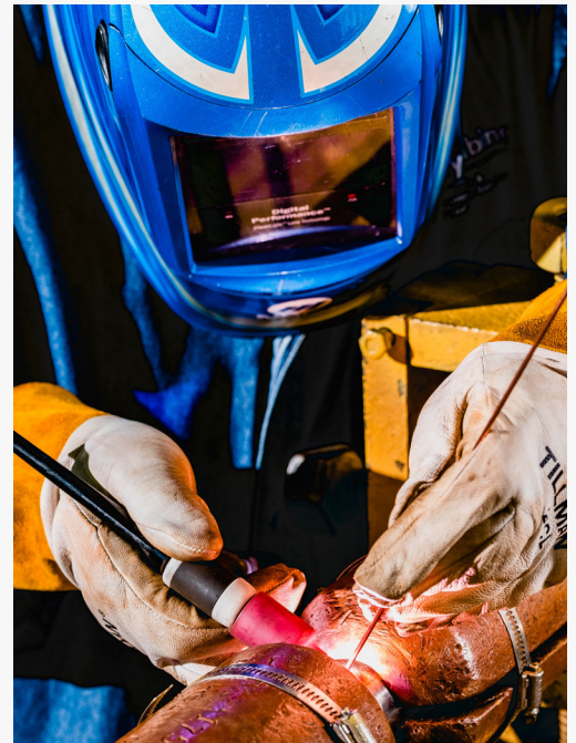
Field-deployable welding procedures for ATP product line
