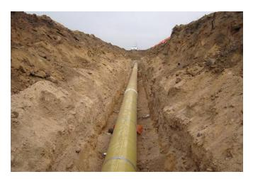
Application: 97% CO<sub>2</sub> gas gathering lines installed in 1993 in New Mexico
