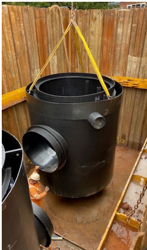
HDPE manhole installation supplied with optional shuttering to accept concrete poured surround.
