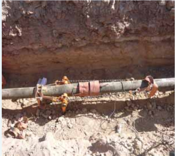
Heat Cured Epoxy Joint
