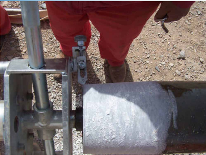
Taper Male Joint Preparation
