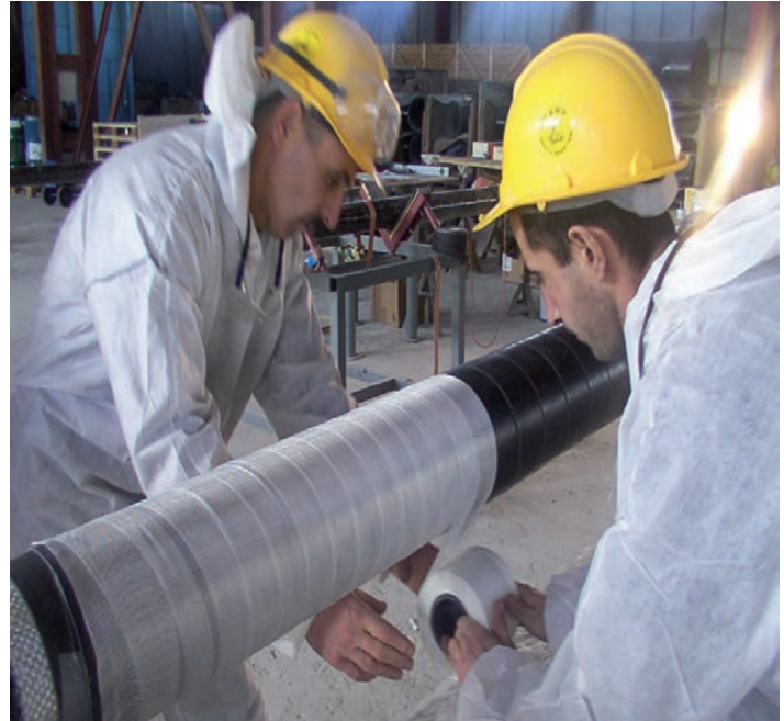
Over-wrapping of Fire Protected Spool with Boat Tape
