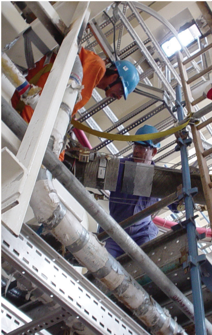
Field Joint of Pipe Spools
