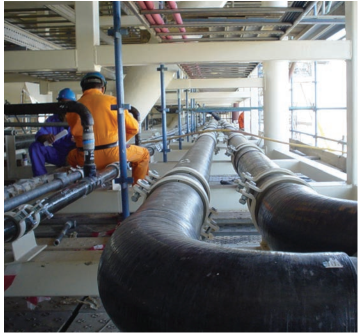
Installation of Bondstrand Seawater Line
