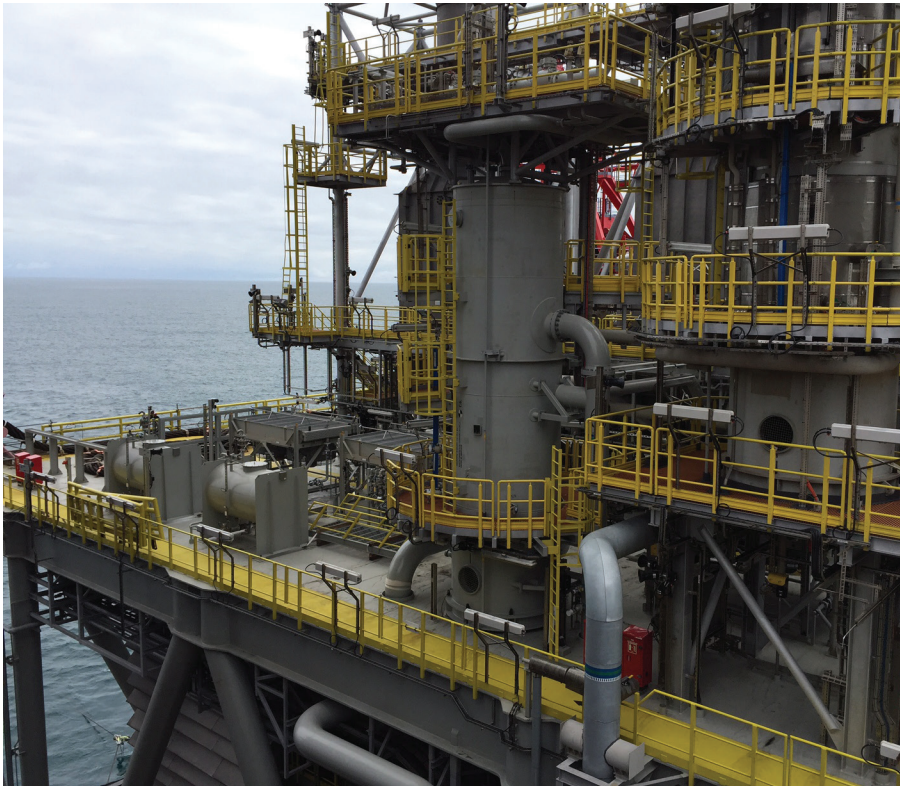
Fiber Glass Systems advanced composite solutions installed on BP Clair Ridge.
