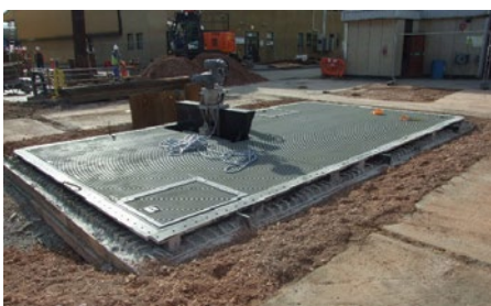
Chamber with optional flow control activated penstock and walkway cover or odour control cover
