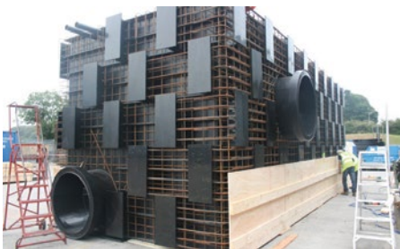
Factory fitted rebar reinforcement and shuttering
