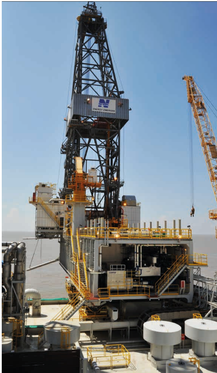
The CJ46 X-Y cantilever and NOV drilling package offer a 1,500,000 hook load capacity, 70 ft longitudinal and 40 ft transverse drilling envelope.
