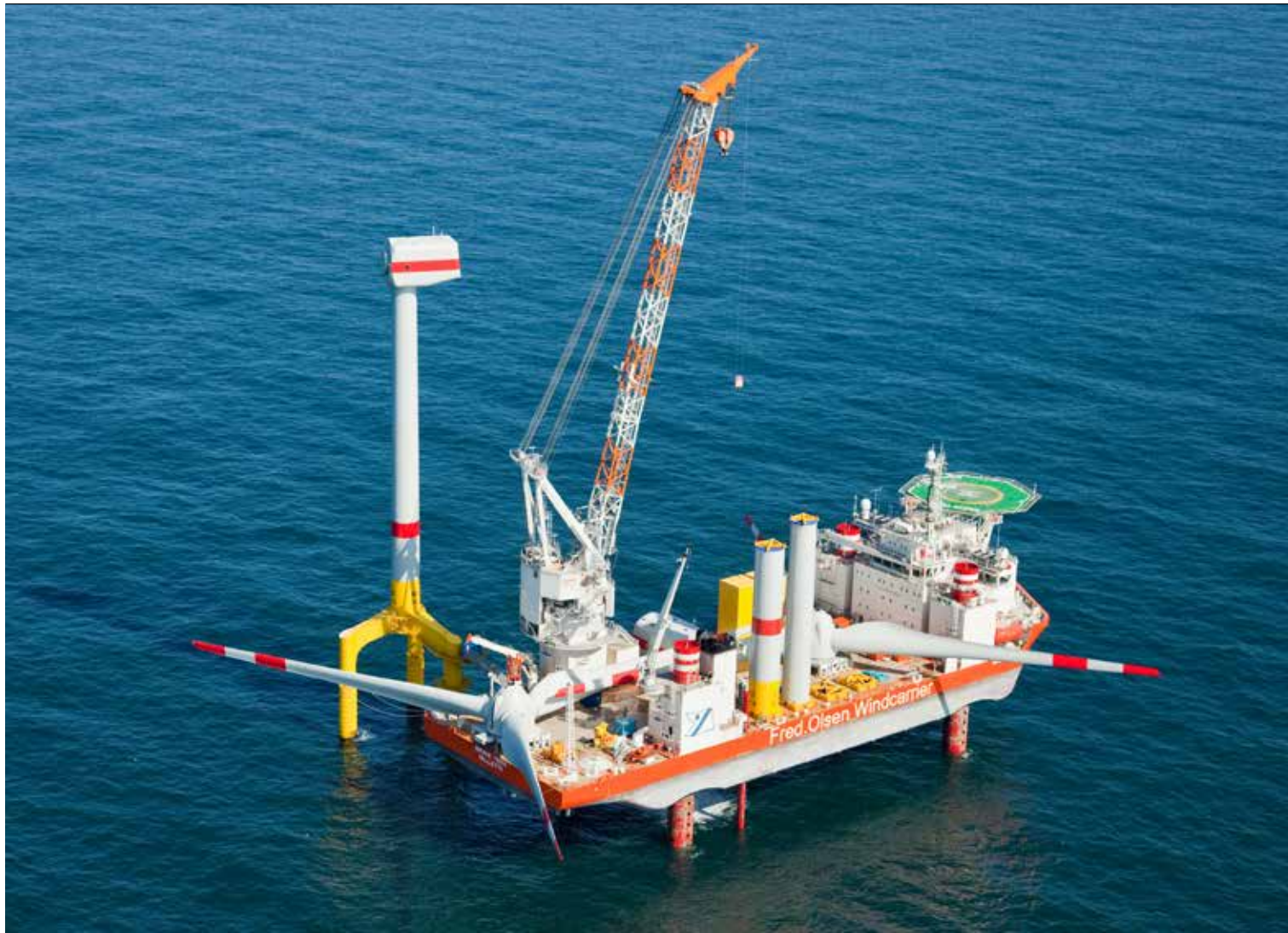
Fred. Olsen Windcarrier's Brave Tern installing wind turbines on the Bard Offshore 1 wind farm, located 100 kilometres (62 mi) northwest of the isle Borkum in 40m (130 ft) deep water (2013).
