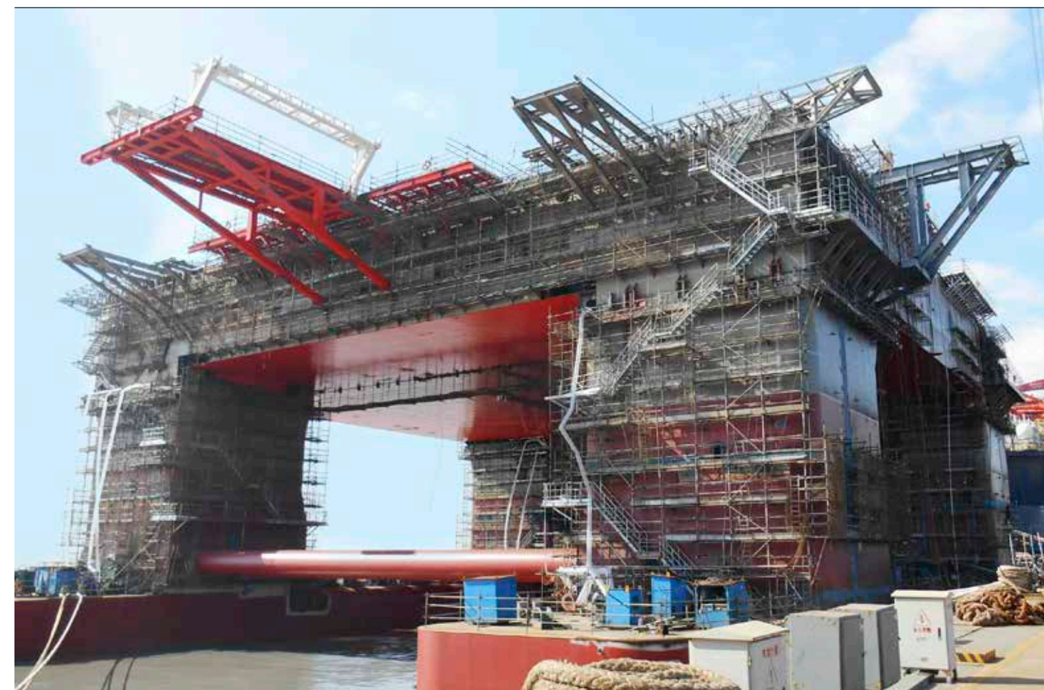
OCEAN500 under construction at COSCO Qidong shipyard
