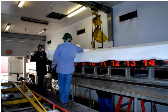
Figure 4 Insulation Layer Being Placed over uPole
