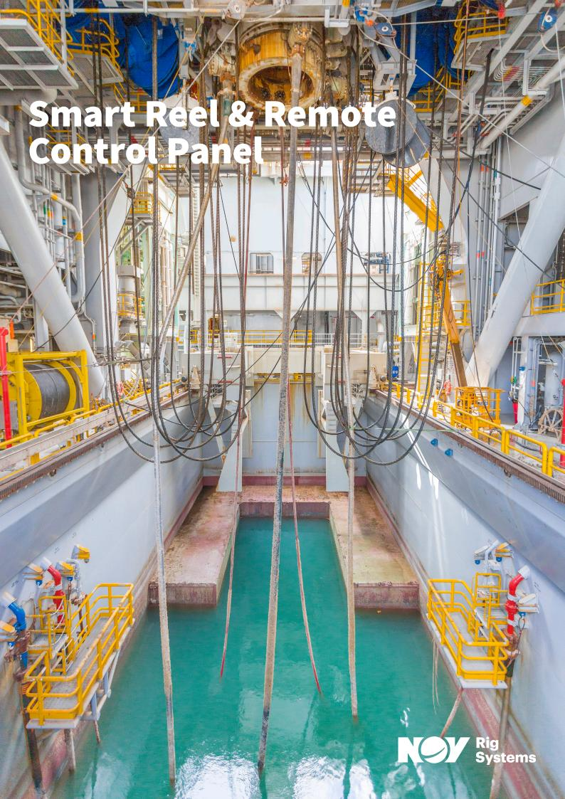
Radoil's Smart Reel provides automated constant tension during stack deployment and retrieval, significantly reducing the risk of umbilical damage.
