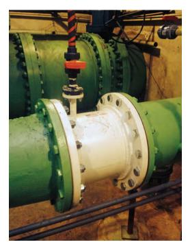
The versatility of Kenics static mixers allows customers to design around existing pipe layout
