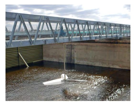
XE-3 impeller installed in a wastewater treatment facility in the United Kingdom
