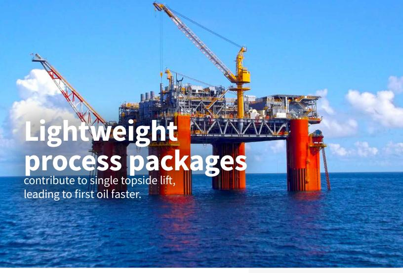
The Delta House deepwater floating production system (FPS) supports three Gulf of Mexico, Mississippi Canyon fields with reservoirs from 12,000 to 18,500 feet. The FPS nameplate processing capacity of 80,000 BOPD, 200 MMSCFD of gas, and 40,000 BWPD required an extensive custom topsides design.
