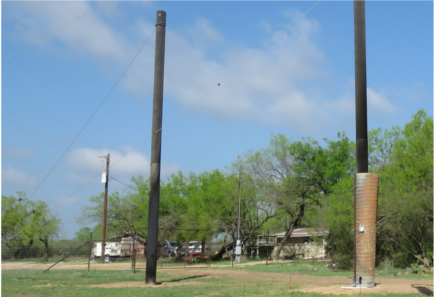
Post-fire test enhanced Ameron uPole, 2-minute exposure
