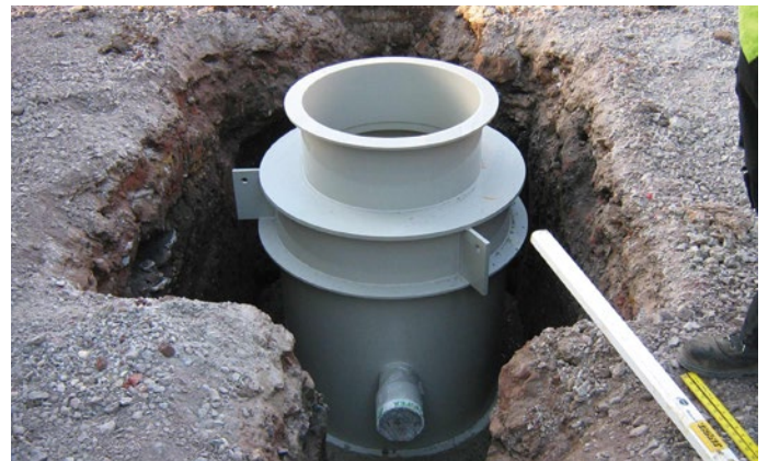
Access turrets are adjustable to suit onsite cover level
