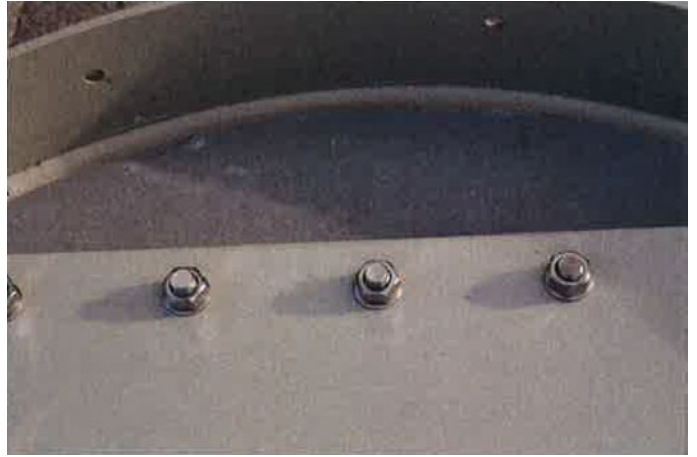
Stainless Steel bolted cover plates with gasket seal
