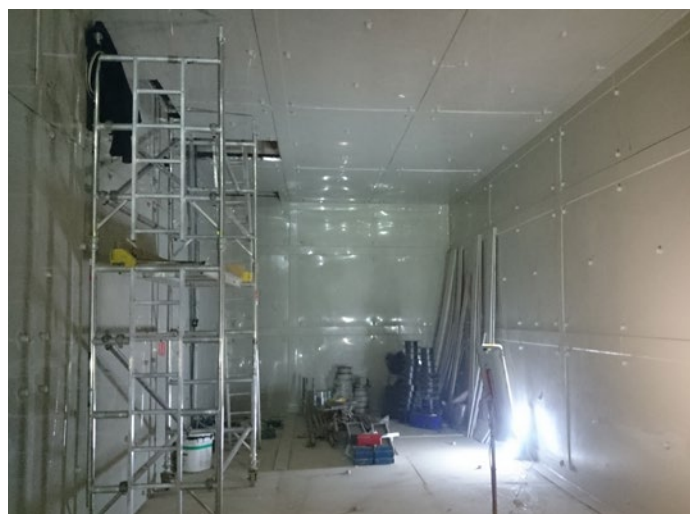
Installation of Pipex Structural Liner
