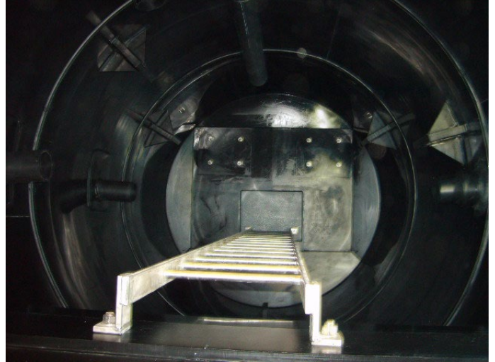
Pump Station with Pipex HDPE Liner installed
