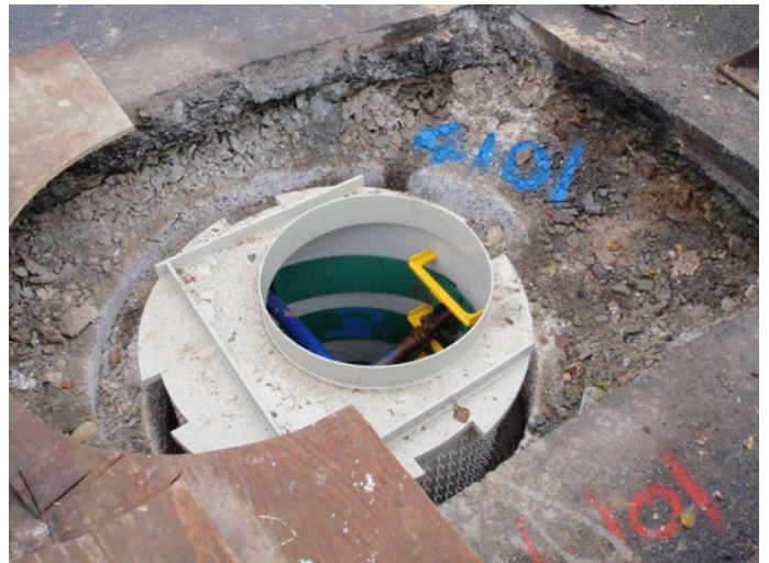
Installation of Pipex Manhole Liner
