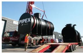
Where required holding tanks can be supplied in sections for site assembly and welding by our site installation team.
