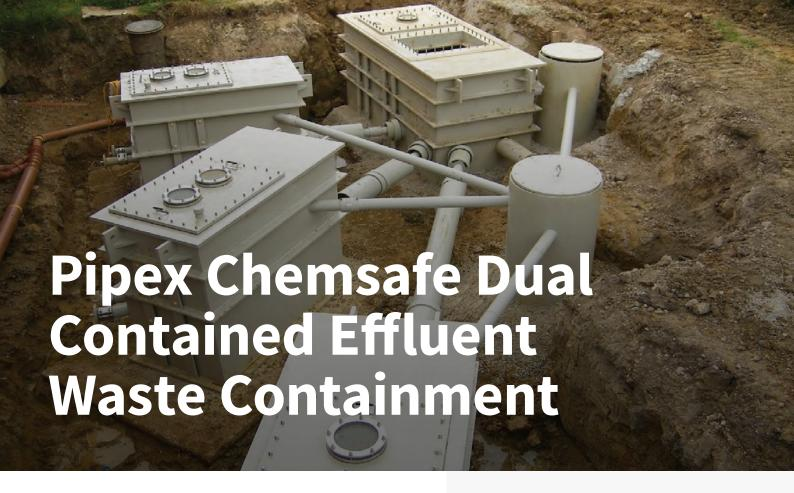
The Pipex Chemsafe™ Dual Contained Pipework and chambers systems is available in for the safe transmission and containment bio-hazardous fluids within high security containment laboratories, chemical/corrosive chemical waste effluent associated with industrial, pharmaceutical and animal research applications for below and above ground applications.
